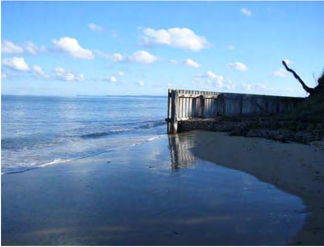
Eastern end of sea wall at approx MHT (June 2007)
